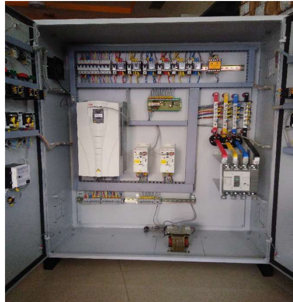
VFD Control Panel
